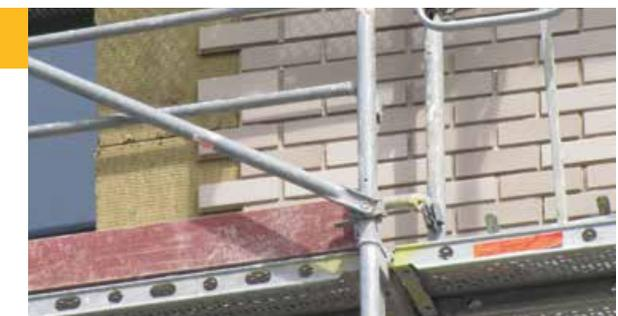
VETABRIC: PREFABRICATED DETACHABLE INSULATING WALL PANELS
